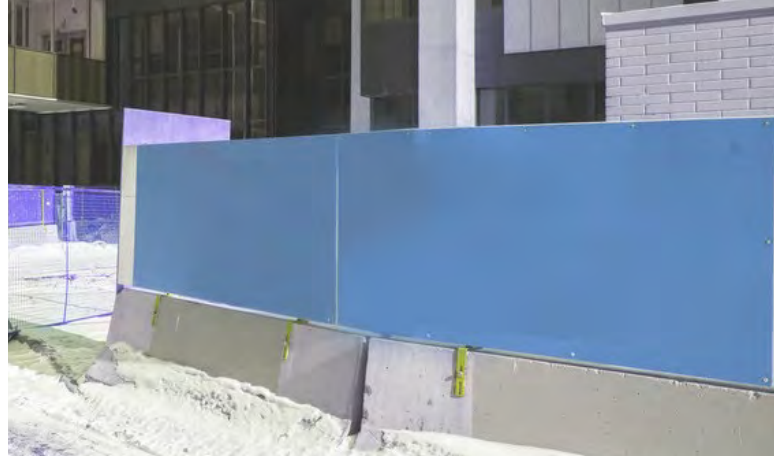
A. Rigid panel mounted to concrete barriers
