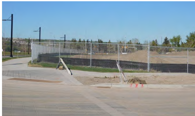
B. Chain link fencing
