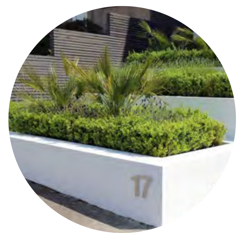
TIRED WALLS; CAST IN PLACE CONCRETE (NATURAL GREY COLOUR) FACING PUBLIC REALM; PLANTED WITH MIX OF EVERGREEN/DECIDUOUS SHRUBS & PERENNIALS
