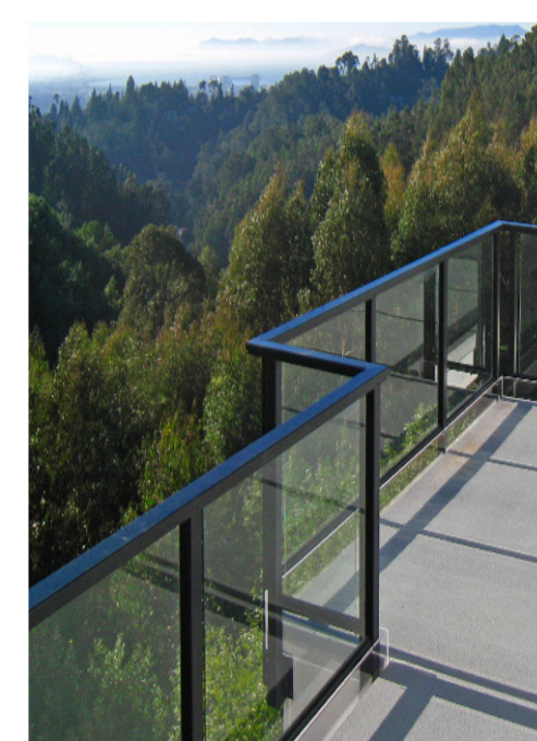
ALUMINUM/GLASS GUARDRAIL COLOUR: BLACK / CLEAR
