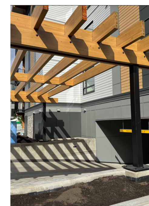
WOOD GLULAM TRELLIS STAINED, COLOUR: TBD
