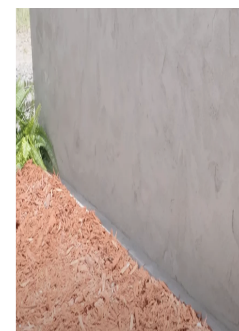
CONCRETE WALL FINISH: SAC RUB LOCATION: RETAINING & PLANTER WALLS
